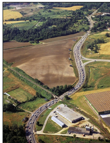
The curve at the RR underpass on Lindbergh (dashed magenta line) was straightened in the 1950s. Photo unsourced.
