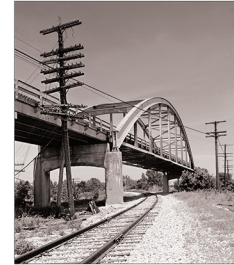
1939 RR Bridge (arrow at left). Historic American Engineering Record
