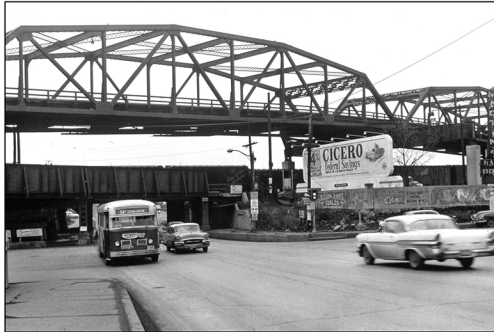
1950s photo of the 1938 RR overpasses for US 66 in Cicero. View is looking south on Cicero Ave. The crossing street is 25th Place.
