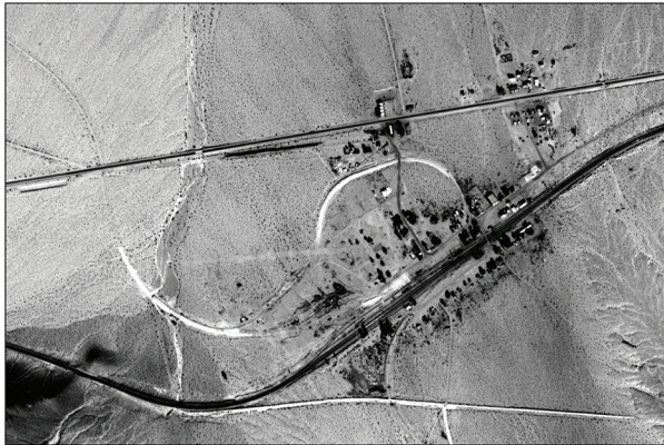
1953 aerial view of Ludlow showing Main St. (green route) paralleling the RR (right side of photo), with many buildings still standing. Angling across the top of the image is the 1931 uniformly paved red route.
