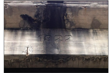
San Gabriel River Bridge. Ian Bowen Photo.
