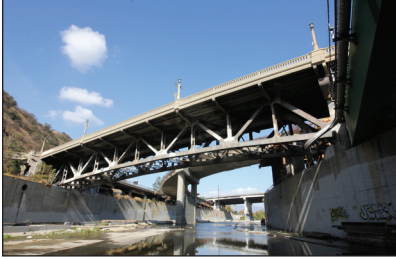
1939 Figueroa St. Bridge (2013)
