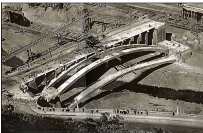
Demo of 127 bridge. City of L.A. Archives
