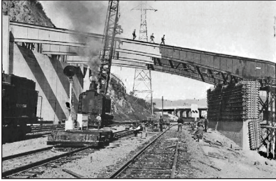
California Highway & Public Works
