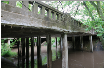
2012 Abandoned westbound bridge
