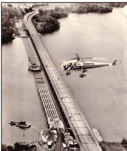
1932 Lake Springfield Bridge (right side of photo) and 1967 EB I-55 bridge under construction
