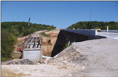
1952 WB river bridge during demolition
