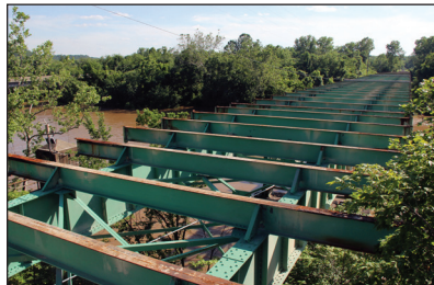
2013 view of the 1933 bridge
