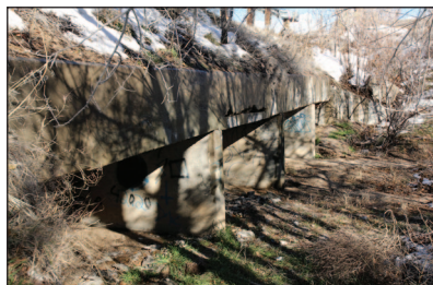
2013 (built when road was widened)
