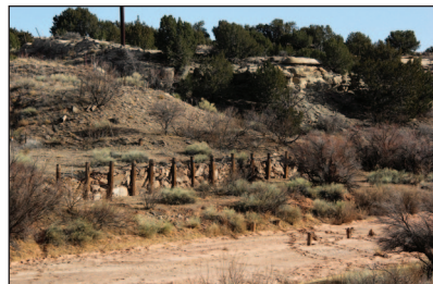
2013 (remains of earlier bridge)
