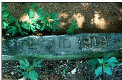
1993 (culvert dated 1919; now buried)
