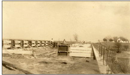
ODOT photo during 1933 construction
