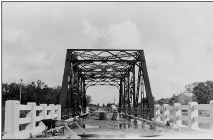
ODOT photo of 1928 bridge
