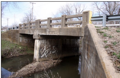
1941 bridge on 1st St. in Chelsea (2013 photo)
