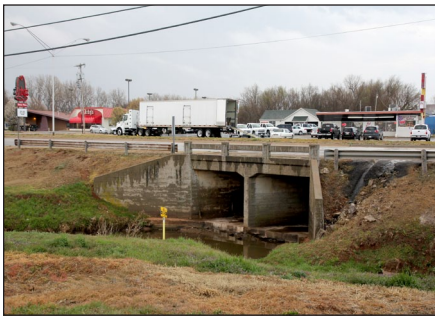
ODOT photo circa 1949 prior to replacement
