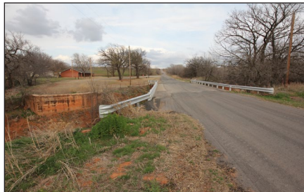
2013 (truss bridge abutments on left)
