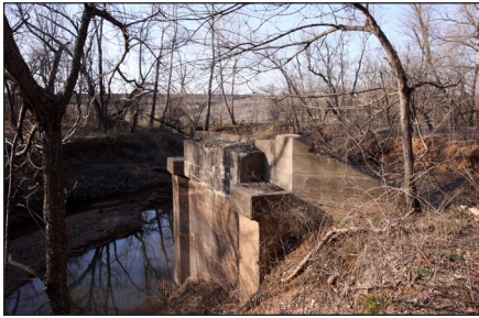
Original site of truss bridge (2008 photo)
