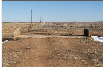
2013 (2nd culvert WB)
