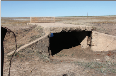
2013 (1st culvert WB)
